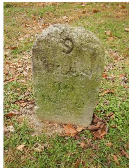
Above: The original sandstone marker at mile 9 on the towpath. Photo by VIP Jim Tomlin.
